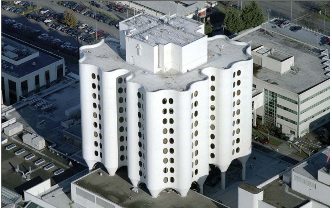
BergerABAM designed the curved-walled concrete nursing tower.
