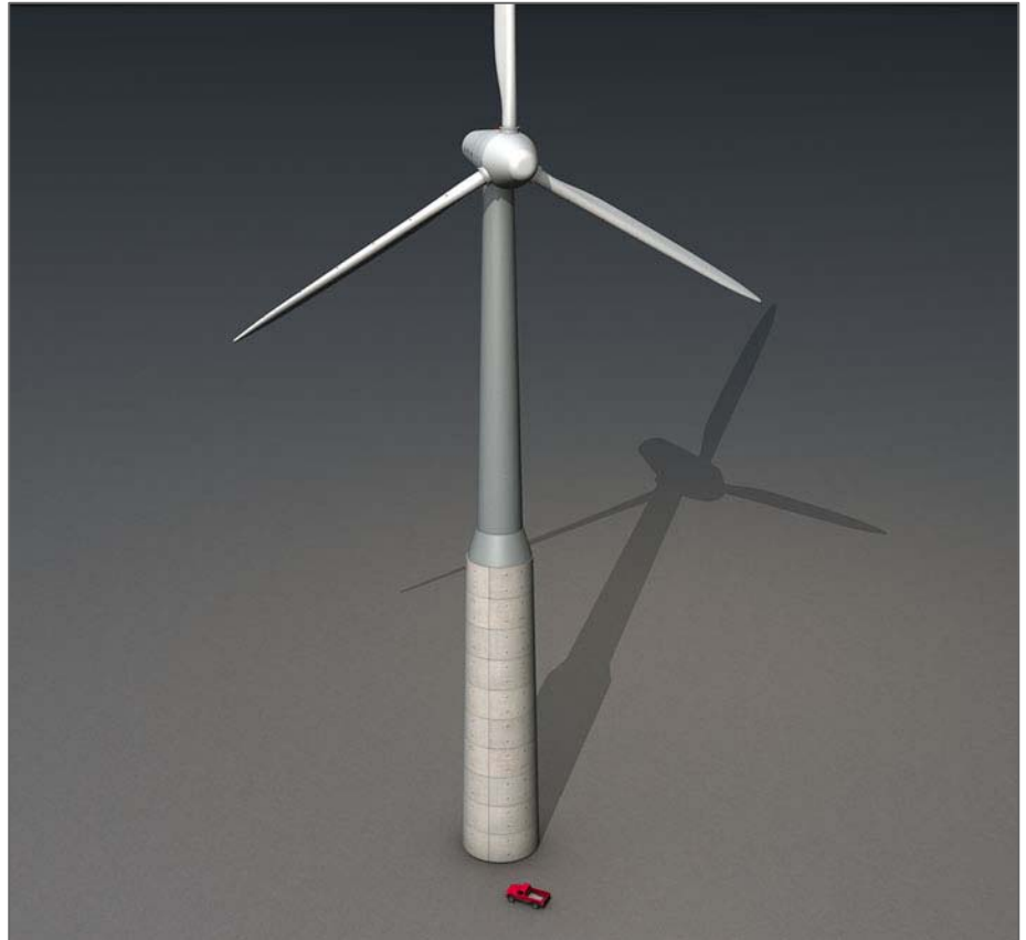
The concrete/steel tower concept was developed to allow installation of the nacelle at the 50-meter elevation and subsequent self-erection to the 100-meter hub height level.
