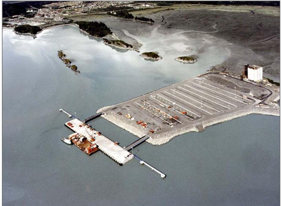
*A first of its kind in the world, the innovative floating container wharf in Valdez, Alaska, designed by BergerABAM was constructed with concrete modules fabricated off site.*
