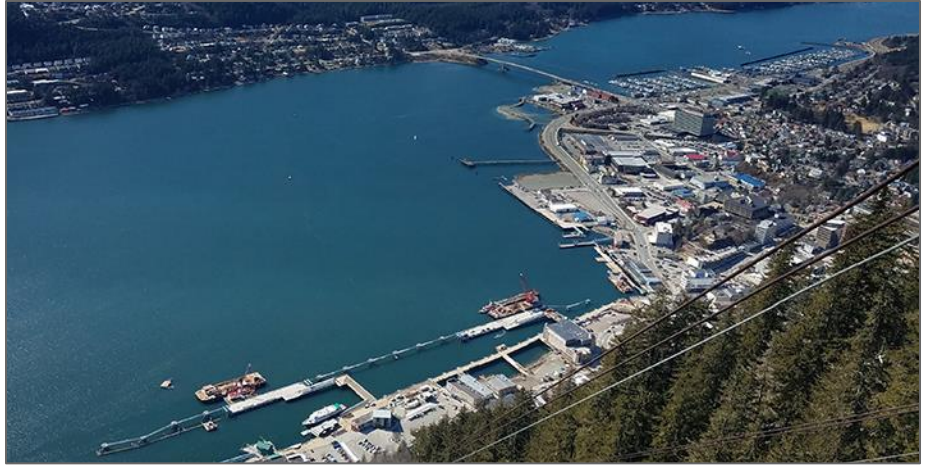
Each pontoon will be held in place by mooring dolphins and accessed from an approach dock by a 140-foot-long transfer bridge. (Photo courtesy of Manson Construction Co.)
