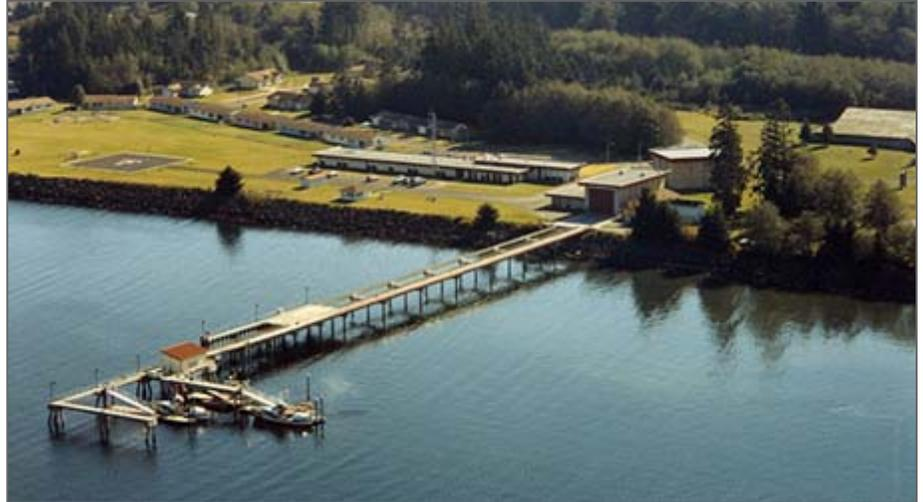
*BergerABAM's marine structure experts developed an innovative framing system to provide resistance to extreme environmental forces while maintaining the economy of a light-duty pier.*
