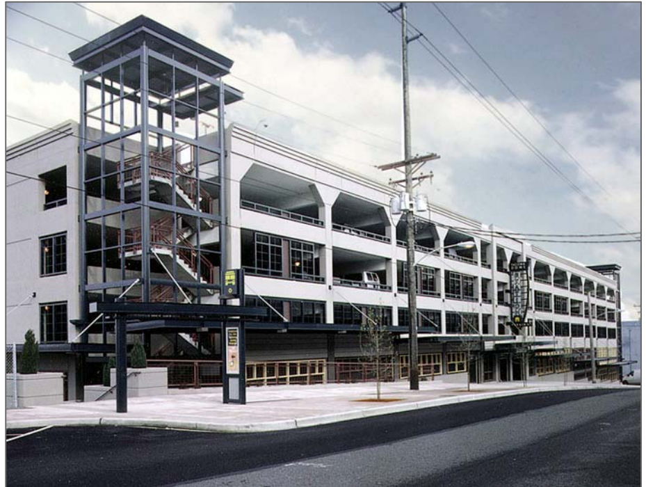
BergerABAM designed the Tacoma Dome Station to accommodate both current needs and future development.
