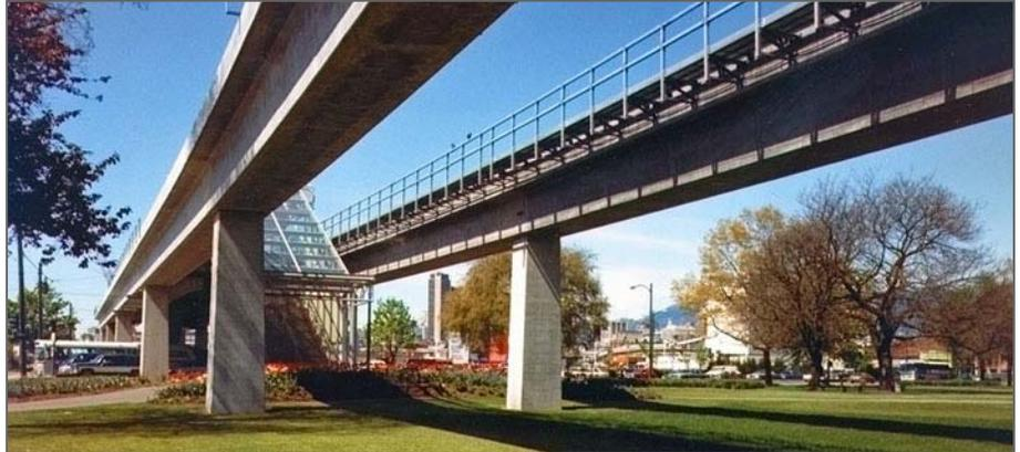
*BergerABAM's conceptual designs were the first steps taken in the actualization of the dual-lane concrete guideway for the SkyTrain.*
