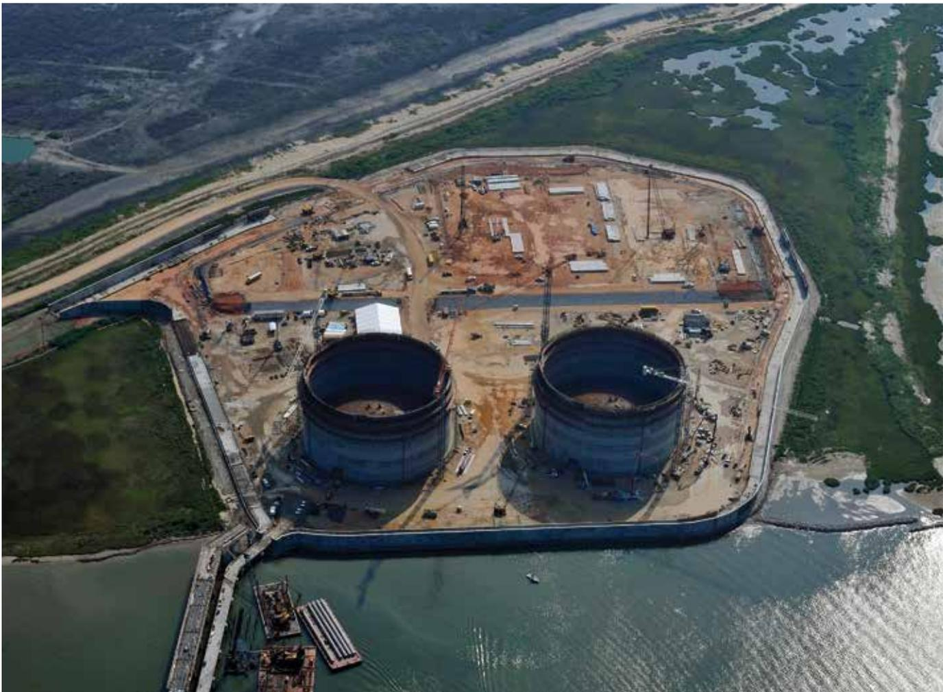
**Figure 1.** A typical liquefied natural gas (LNG) receiving terminal showing the marine berths for the LNG carriers and the LNG storage tanks and associated regasification equipment under construction. The secondary containment roof has not yet been constructed.
