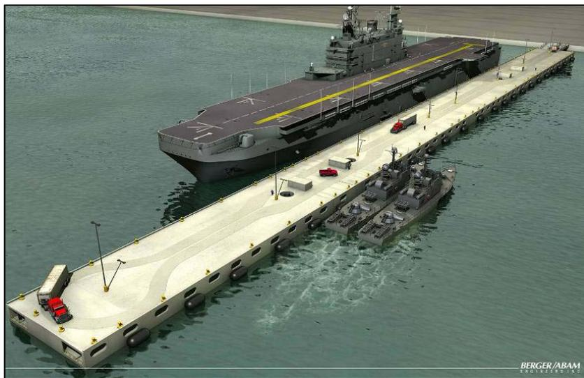
Figure 1. A concept for relocateable Modular Hybrid Pier.
