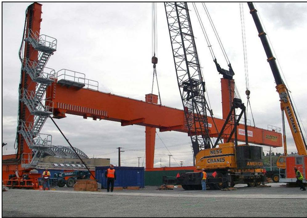
**Figure 7. Erection of rail-mounted gantry crane.**
