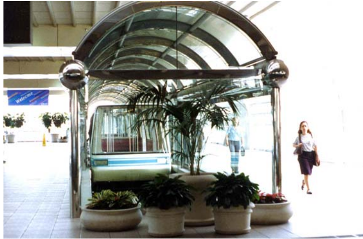
Figure 3. Orlando Airport – APM Station
