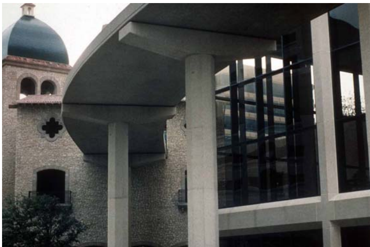
Figure 2. Las Colinas – Clock Tower Station
