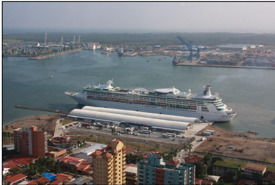
Figure 7. Colón 2000 cruise terminal with second berth completed.
