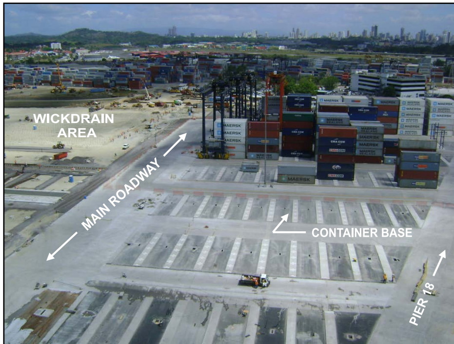
Figure 12. CW1 Yard Construction.
