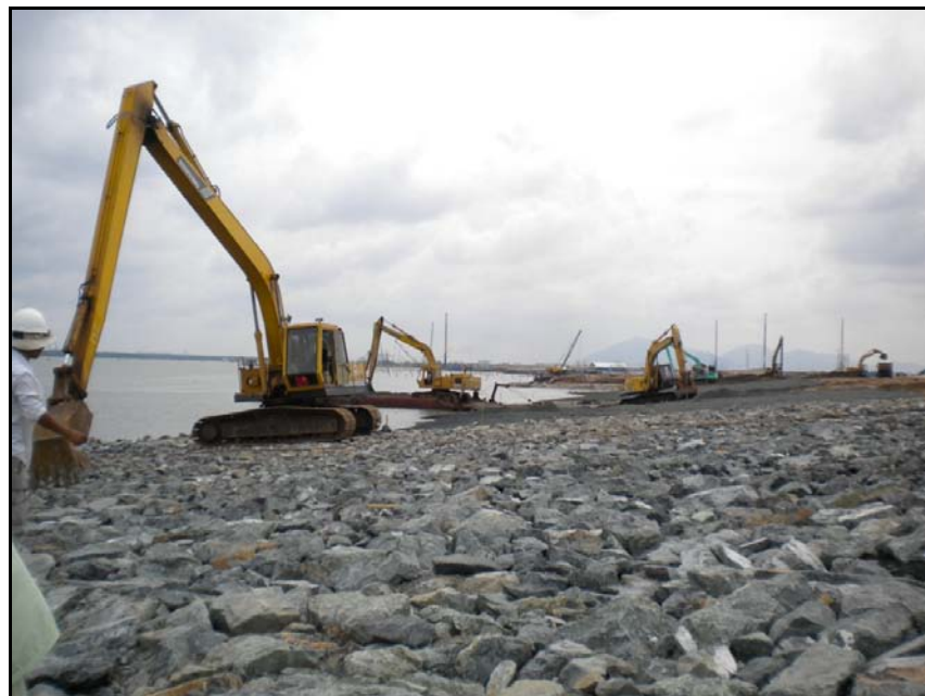
Photo 2. Sloped revetment, June 2009.
