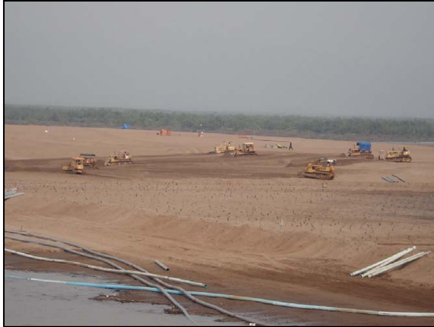
Photo 1. Aerial overview, November 2008.
