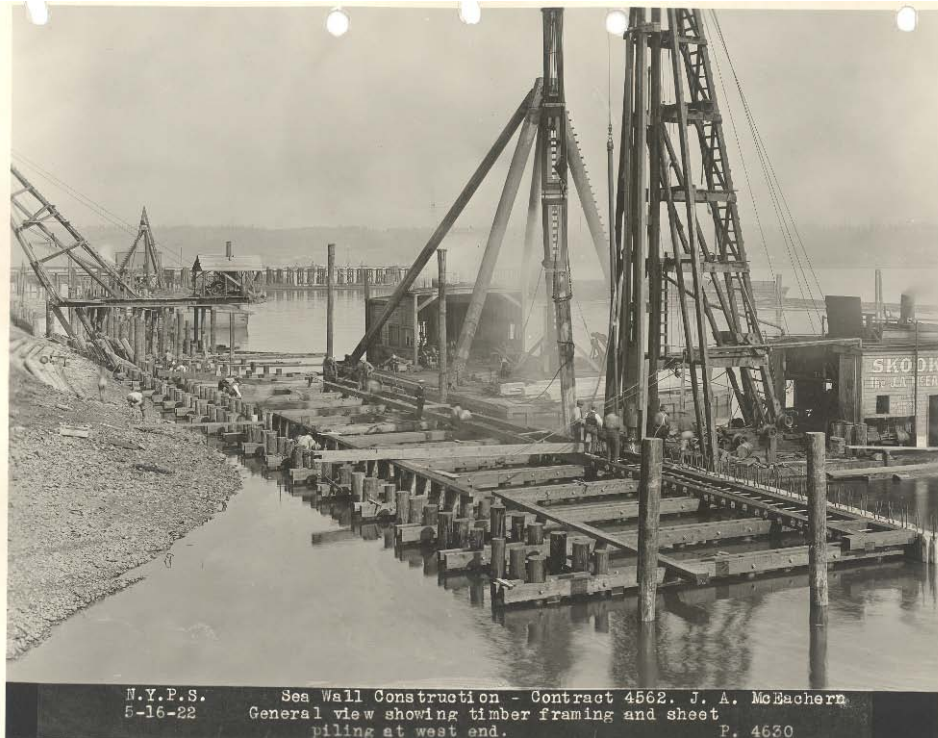
Figure 2. Original quaywall in construction, 1922.
