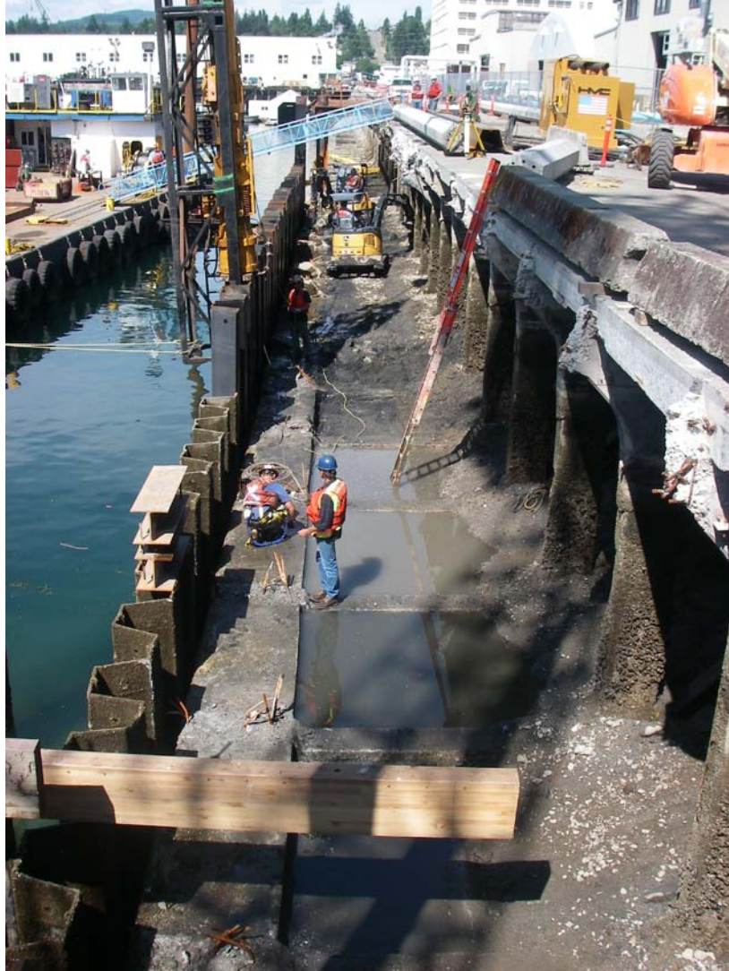
Figure 5. Quaywall 729 driving sheet piles, 2009.
