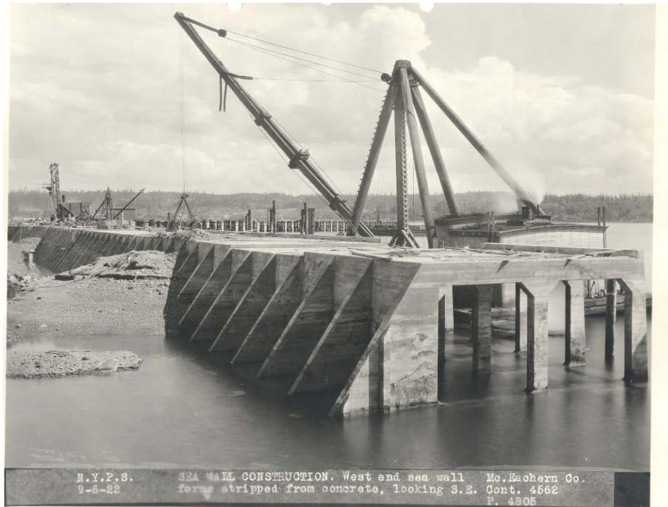
Figure 3. Original quaywall in construction, 1922.
