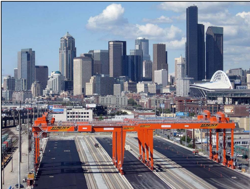
Figure 8. RMGs at Intermodal Yard.
