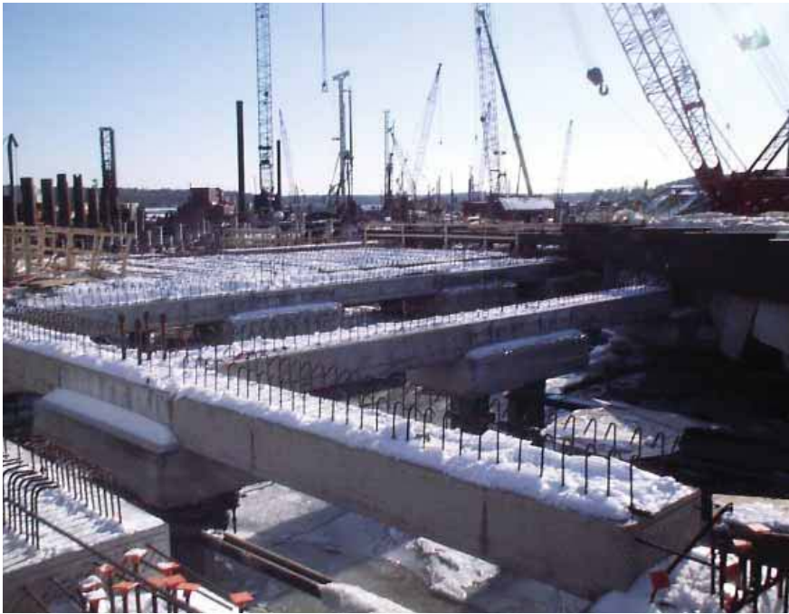
Fig. 3. Coastal Maine in winter presents harsh weather conditions for marine construction. The average low temperature for December in coastal Maine is about 15 F (-10 C). Photo courtesy: Guy F. Atkinson Construction Company.
