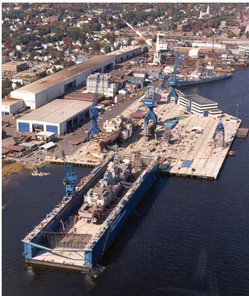
Fig. 2. Aerial photo (looking north) of the completed shipyard expanded facilities in operation. Photo courtesy: Bath Iron Works.
