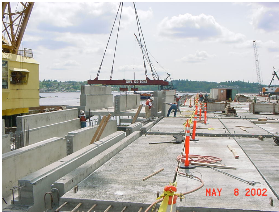
Figure 4: View of Precast Concrete Utility Tunnel Being Erected
