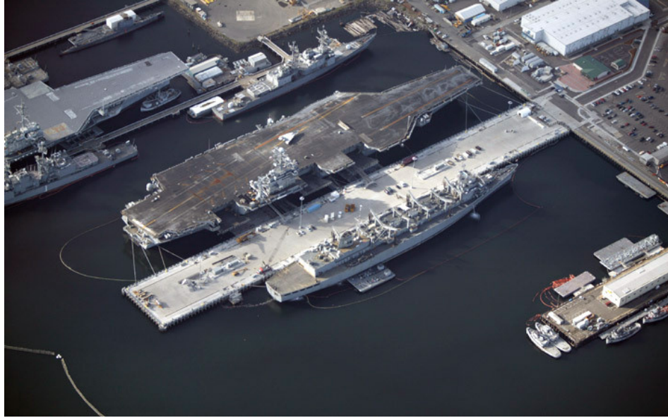
Figure 1: Completed Pier Delta
